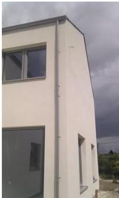
**Fascia / Soffit** - there is none like in many traditional house, the fascia / soffit we are used to seeing is apparently an import from the UK British Standards transposed in the 1960s. Regardless, you need to have this understood as the start of the build so that this is allowed for, its too late to decide half way through.
