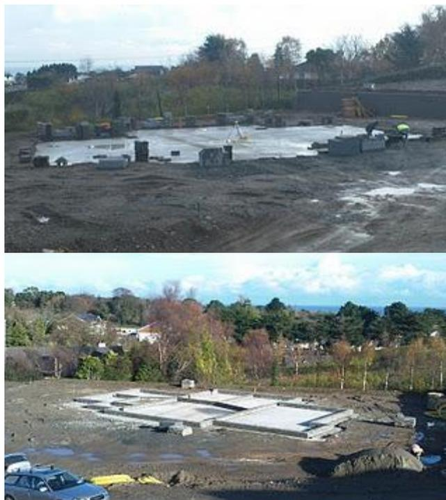
Rising walls going in on the slab; radon layer, timber frame & insulation are next. Started putting plants down on site too - its the time of year to plant those daffodils & we had received a large consignment of them.
