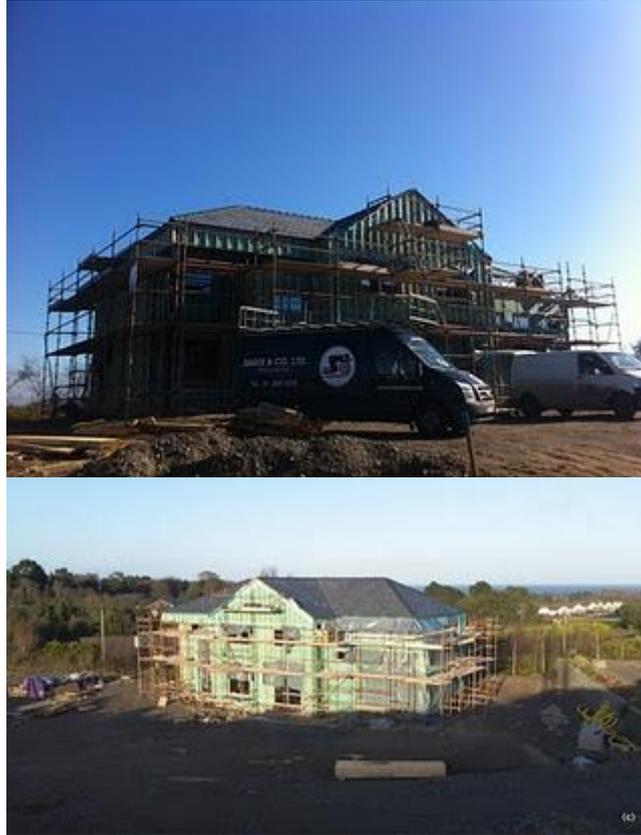
Pace on the build has really increased in the last week. The roof is now fully complete & the exterior board (no block!) is going up on the outside. The board which sits proud of the building by approx 50mm to give a ventilated cavity round the structure will then receive a permanent monochrome render.
