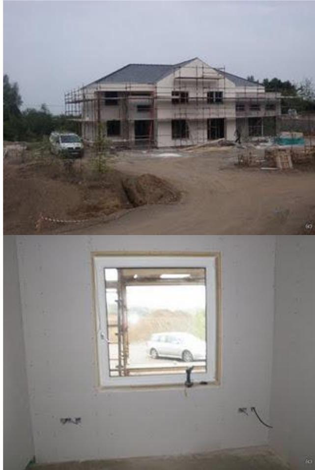
The blower doors test was done to to the Passivhaus standards which means pressurising and depressurising by 50Pascals ( feels like a strong wind when opening & closing doors) and we passed the criterion. Photo below of the fan fitted to an open window for the test.
