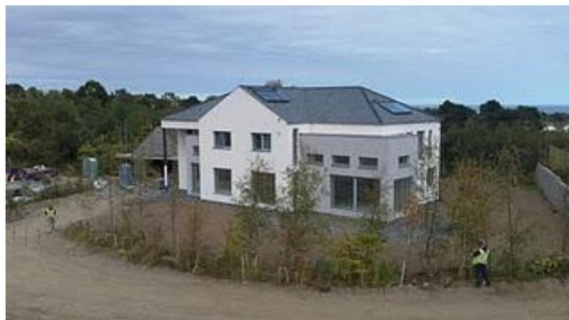
A case in point to the date has been the supply of our monocouche render system by Parex Lanko ( a French company), supplied by REP Ltd. in Ireland as part of our wall buildup. Technically, the outer skin of the building consists of a ventilated cavity battened out out, a 9mm magnesium renderboard which is then coated in an approx
